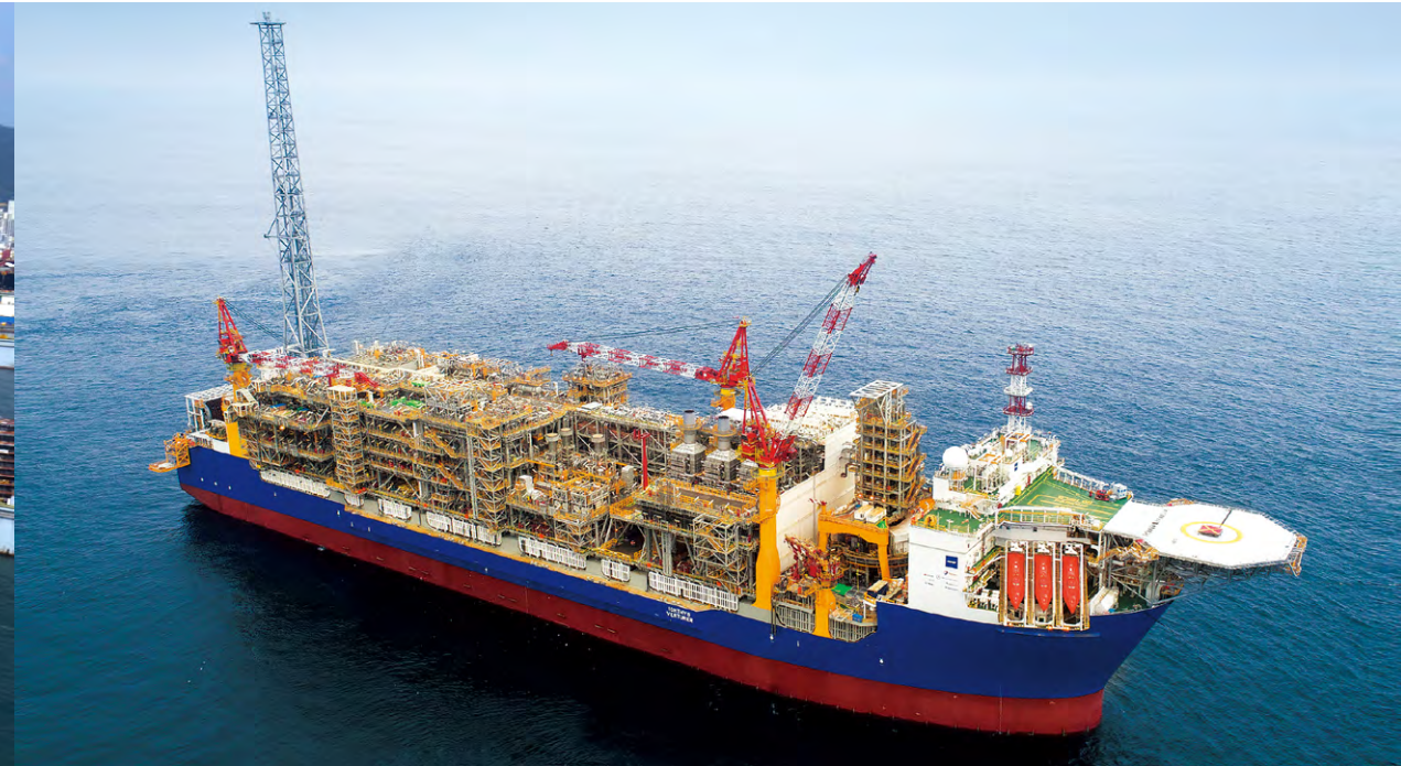
FPSO (Floating Production, Storage, and Offloading)
