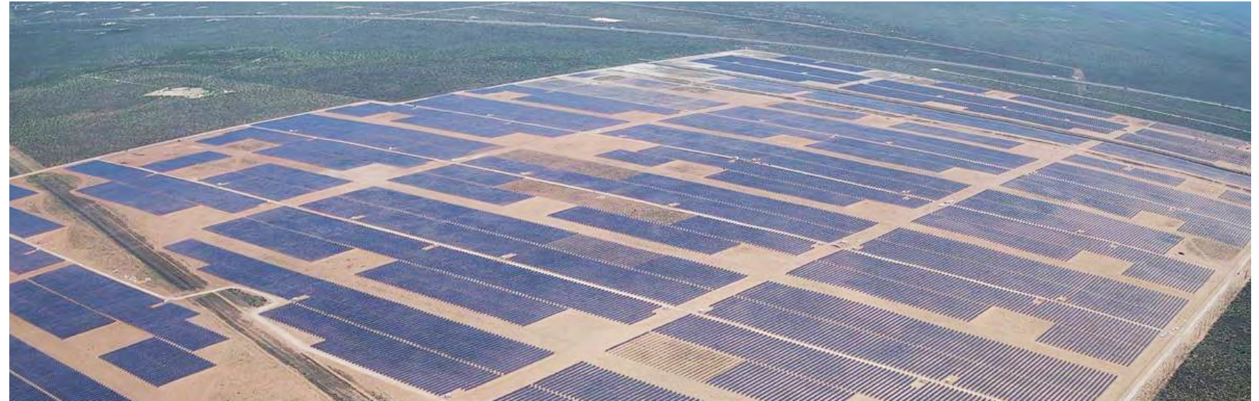
Oberon 1A solar power plant in Texas, US
