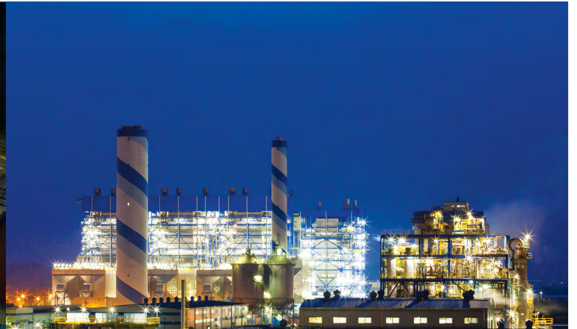
Yeosu cogeneration plant
